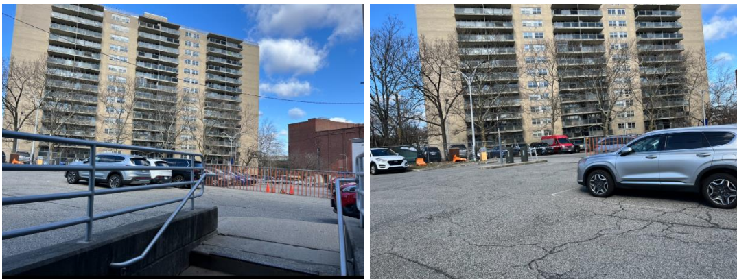
Figure 3 Views of locked parking area with uneven pavement
